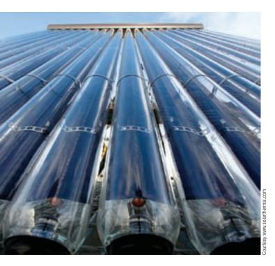
Evacuated tube collectors are more efficient than flat-plate collectors in cloudy or colder conditions, but can be more expensive.
